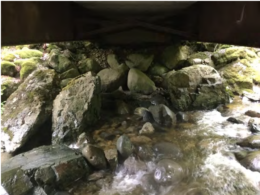
Right Bank Abutment when facing downstream
