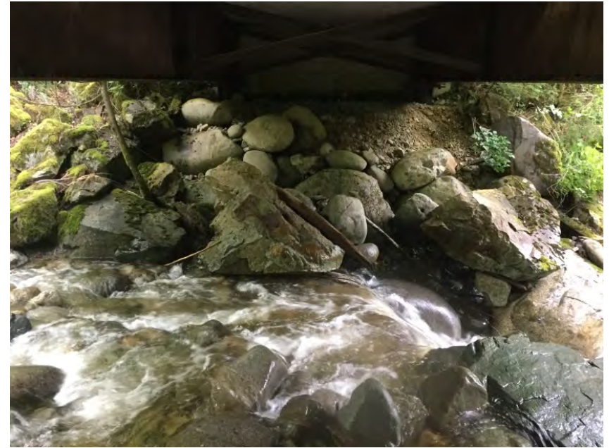
Left Bank Abutment when facing downstream
